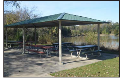
Central Park Fishing Pier Shelter
